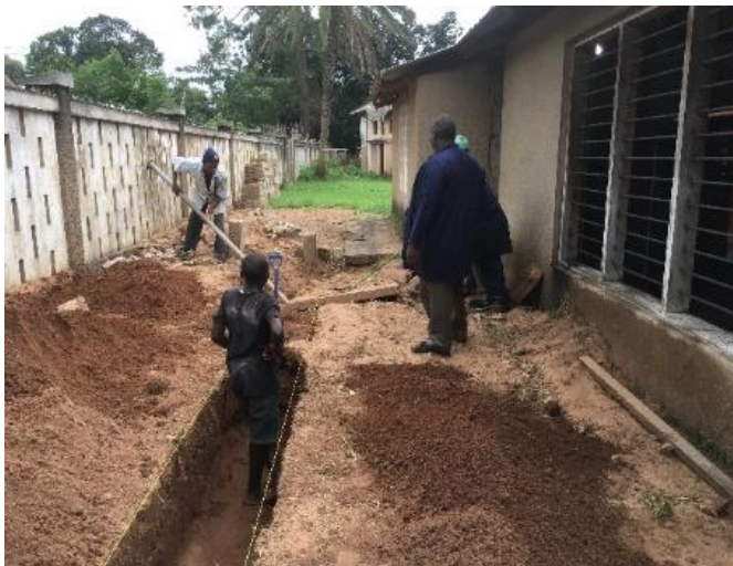
Construction of power back up Batteries Room.
