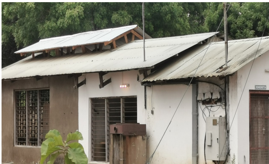
Picture: Improvised Ventilation System on the generator roof to facilitate cooling of the generator
