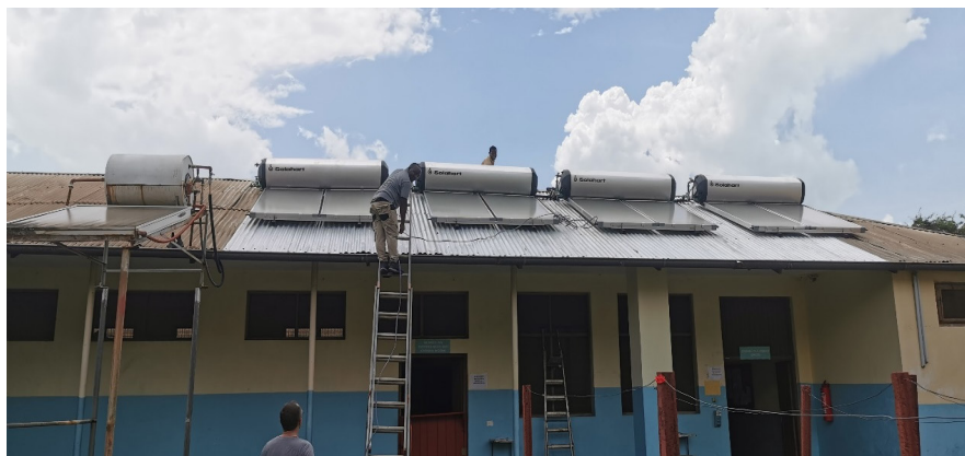
Picture: Solar Heaters 1800lts tanks
